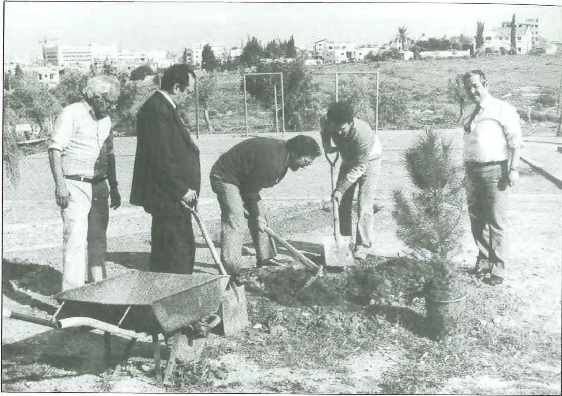
HTI's follow-on contribution to the Strovolos Acropolis Park, the work being overlooked by former Director Dr George Christodoulides.
