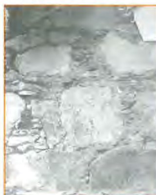
Figure 4. Rubble stone construction of the wall of the church.
