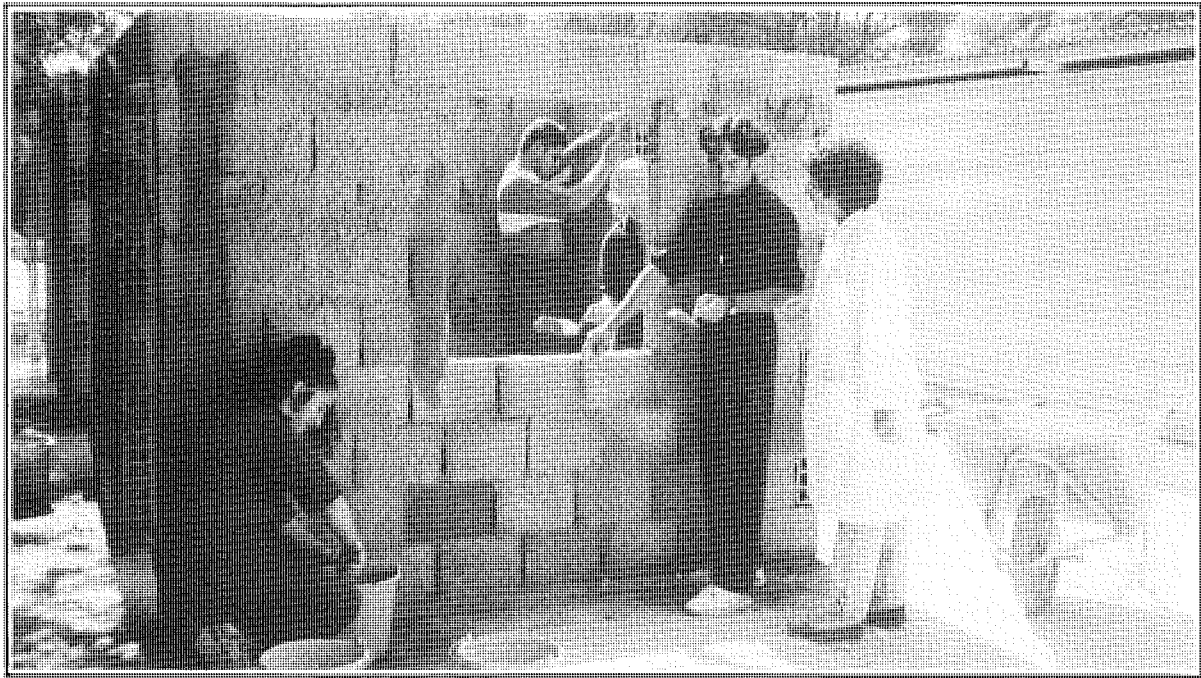
Male and female HTI students during their training in construction works
