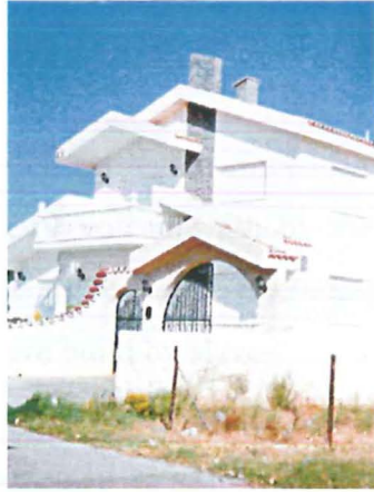
Photo 1: Modern concrete structures
