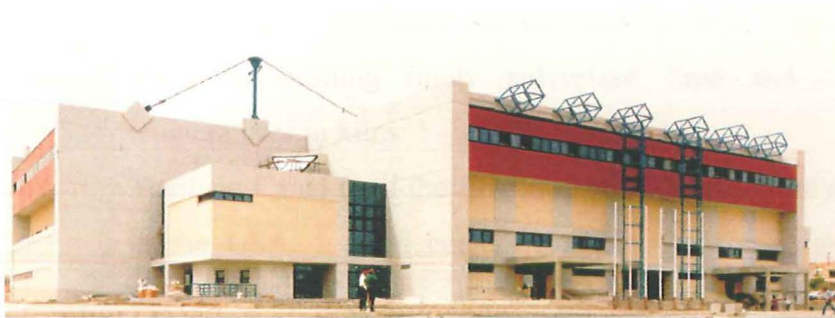
Photo 2: Modern concrete structures
